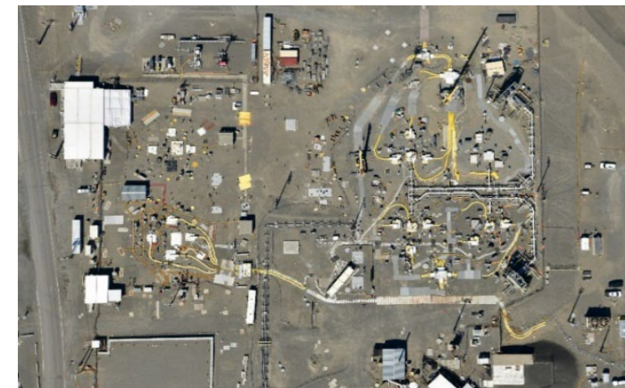
AY Tank Farm (left), AX Tank Farm in Retrieval (right)
