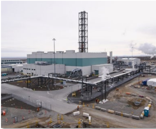
Low-Activity Waste Facility
