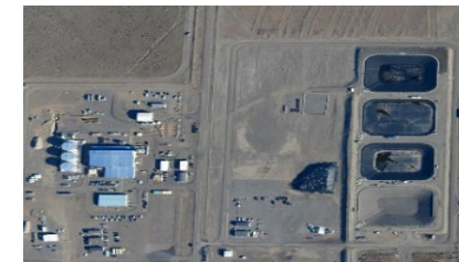
Liquid Effluent Retention Facility Basin and Effluent Treatment Facility
