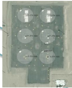
TY Tank Farm Barrier
