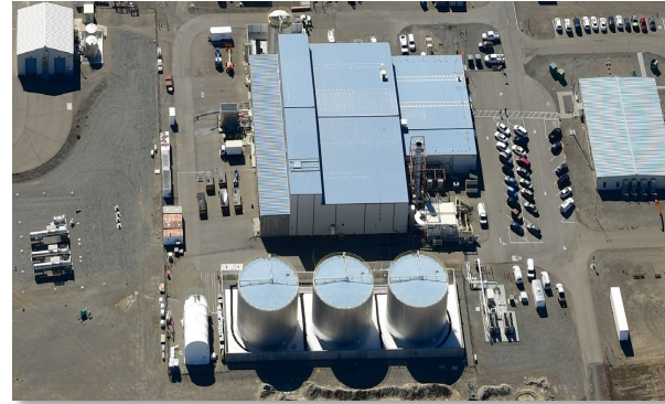
Liquid Effluent Retention Facility/Effluent Treatment Facility
