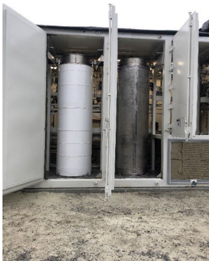
Installing Ion Exchange Columns
